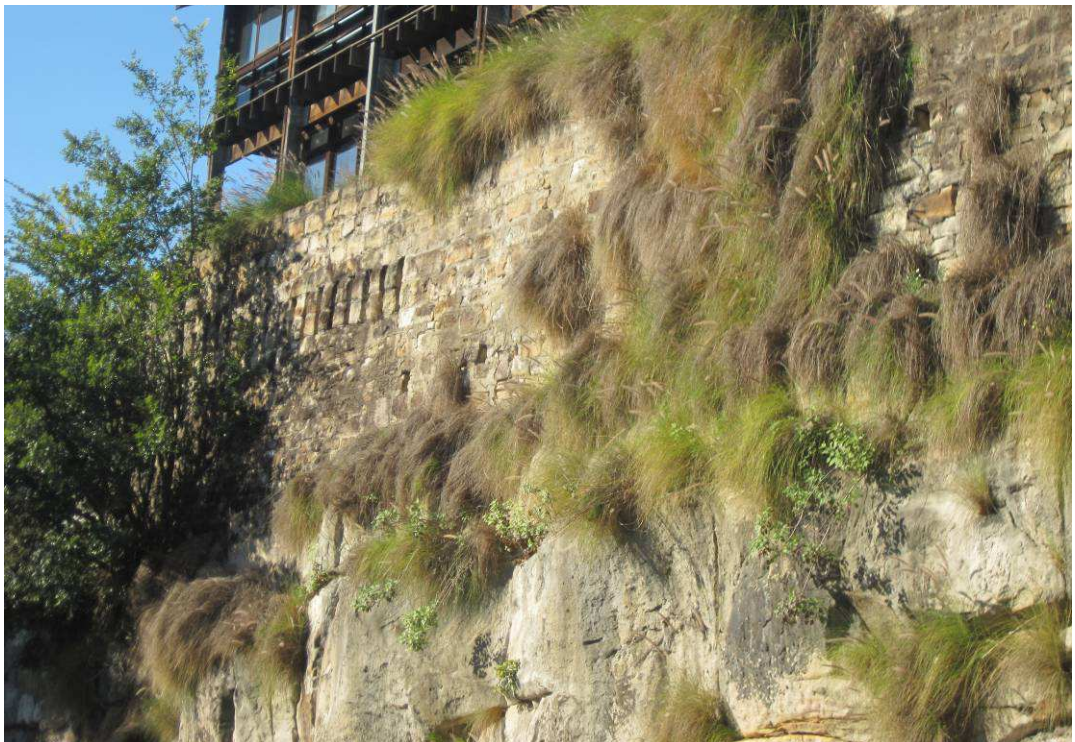
Figure 24 The stone wall above the cliff face at the rear of 153-155 Brougham Street may be the retaining wall for which a building application was lodged during 1923 (City of Sydney Archives BA 466/23). Photograph: Tanner Kibble Denton Architects.
