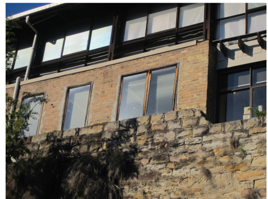
Figure 26 Brick infill at the base of the cliff face, below the swimming pool at the rear of 161-165 Brougham Street (left). The date and reasons for the infill have not been ascertained, but the stone wall on the top of the cliff face (right) may be associated with the garages built during the 1920s at the back of 159 Brougham Street. The common brick wall above the stone wall may be part of the garages; the window openings were formed at some time after 163 Brougham Street was completed. Photographs: Tanner Kibble Denton Architects.
